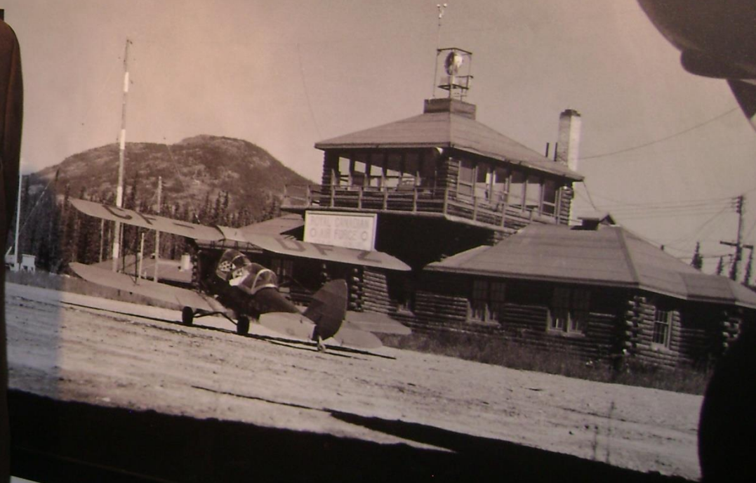
Teslin Airport Control Tower 1952 George Johnston Museum, Don Williams
